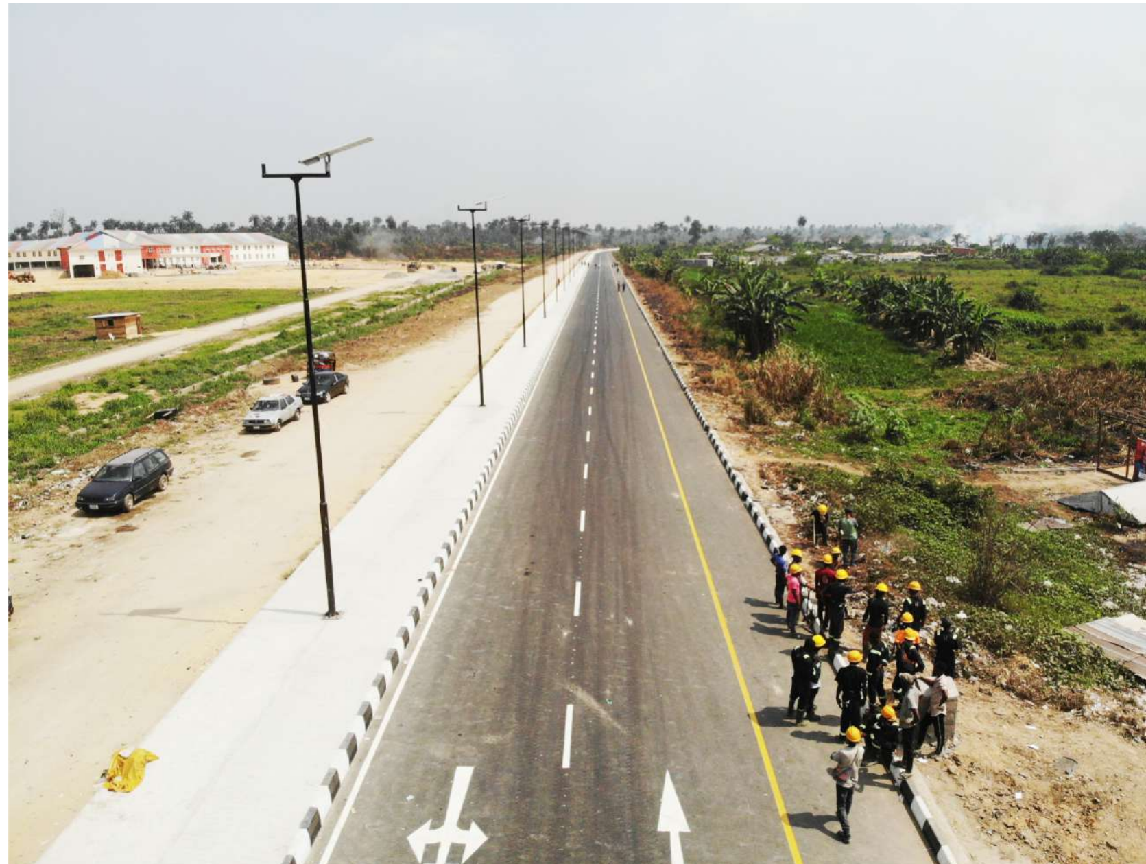
AIT/IGBOGENE ROAD COMPLETED
