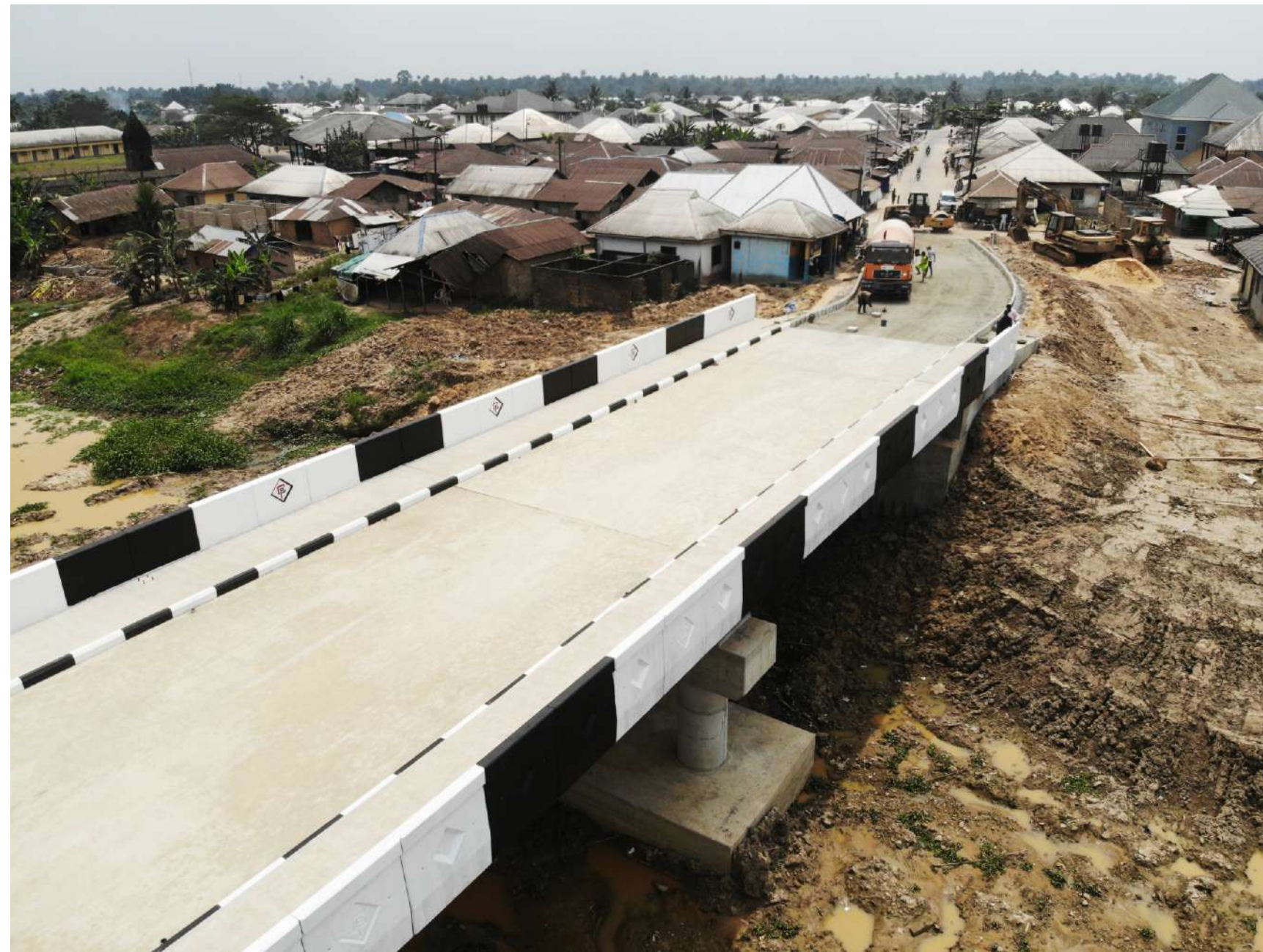
ELEBELE BRIDGE COMPLETED
