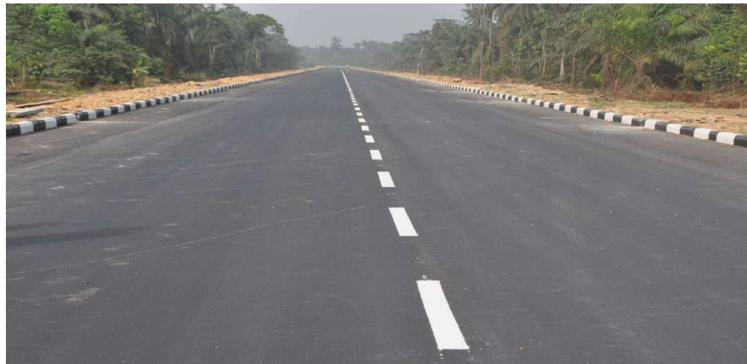
IGBEDI ROAD COMPLETED
